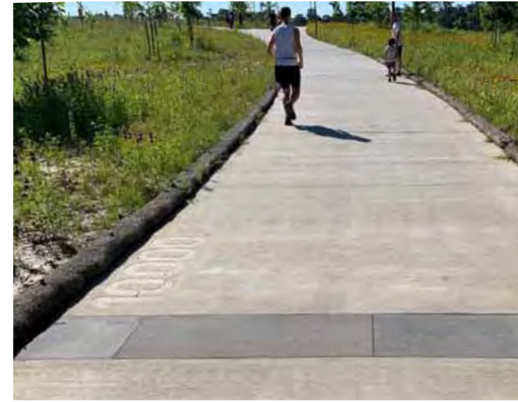
Kinder Land Bridge, Houston, TX Stored Path Materials
