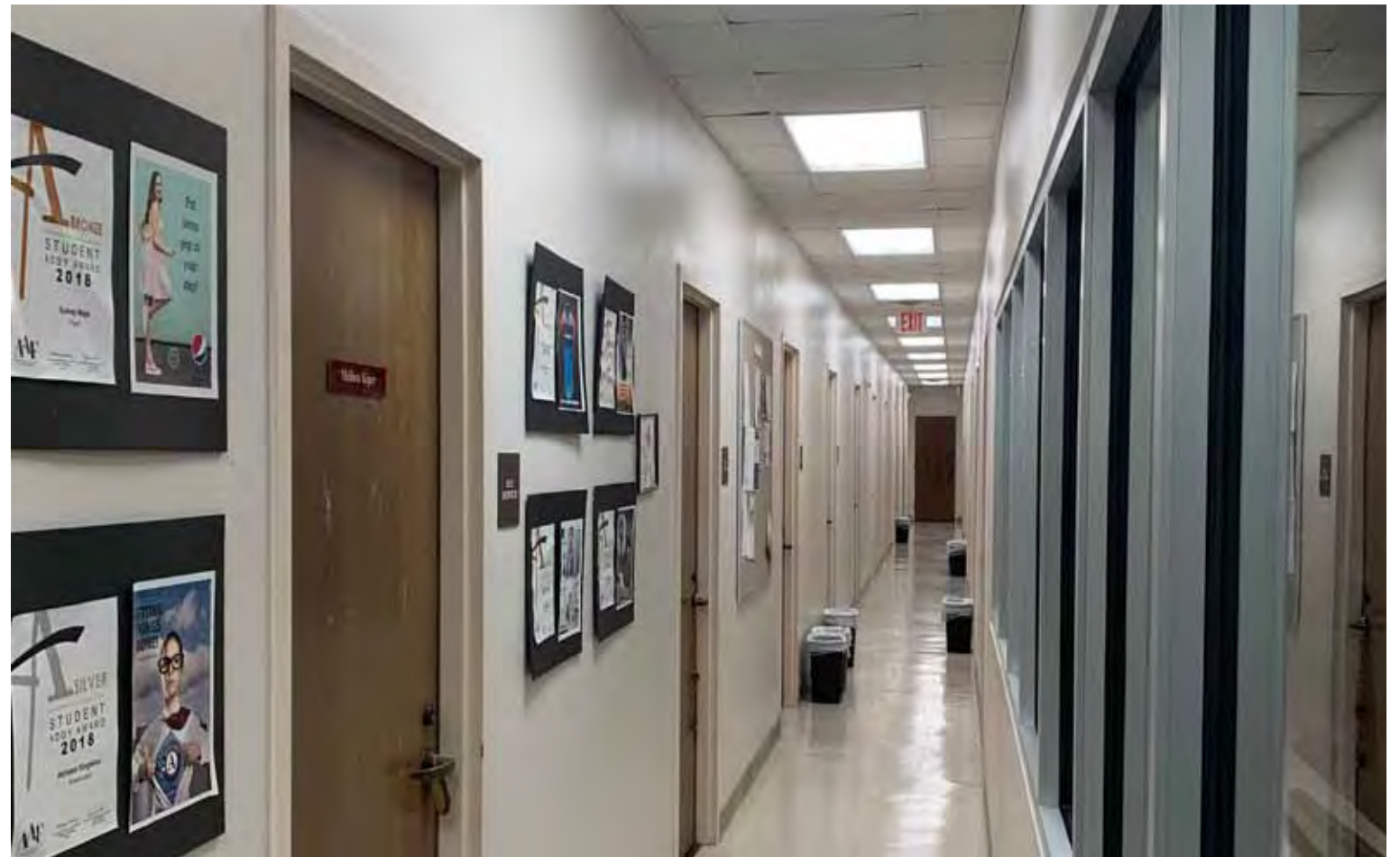
Hallways leading to faculty suites are long and narrow with inadequate natural light
