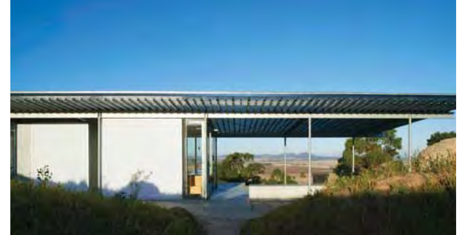
Shack in the Rocks, Victoria, Australia Sean Godsell Architects
