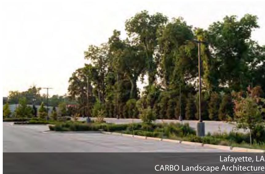
Permeable parking stalls, concrete drive aisle, native plantings CARBO Landscape Architecture
