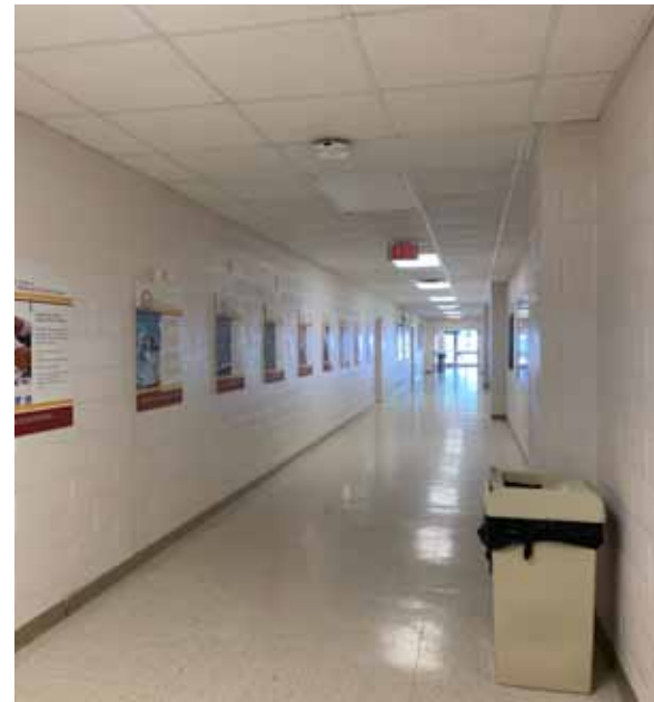
Concrete block walls look institutional
