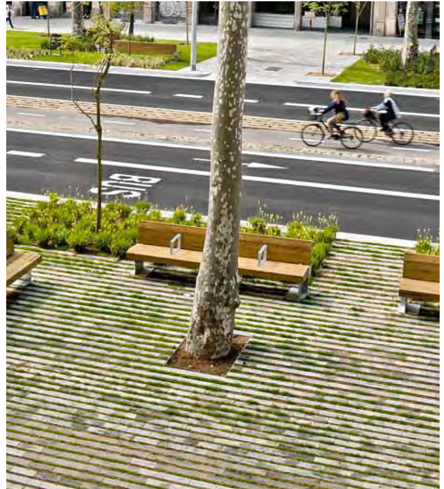
Permeable Paving, Passeig de St. Joan boulevard. Barcelona, Spain Lola Domènech
