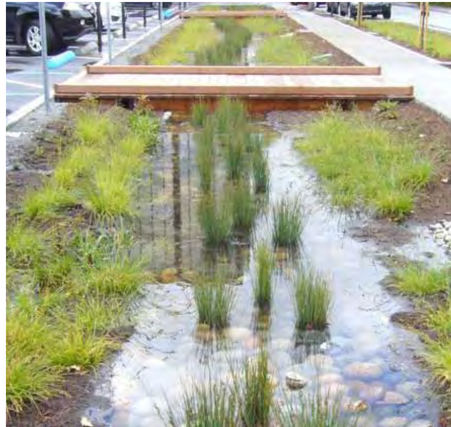
Raingarden at Curb, 21st Street, Paso Robles, CA MIG | SvR
